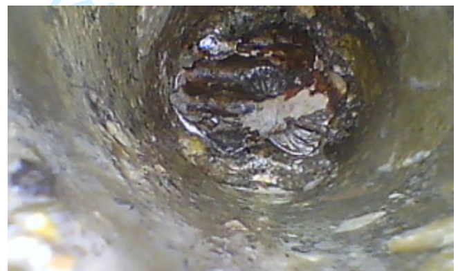
Figure 6 Video-endoscopy to check tendon deterioration.
