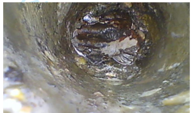
Figure 6 Video-endoscopy to check tendon deterioration.
