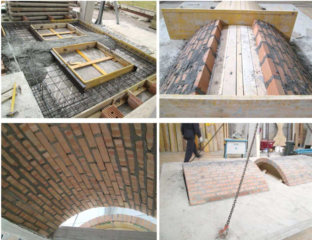
Figure 31 - Sequences of images taken during the construction of V.04.c and V.05.c
