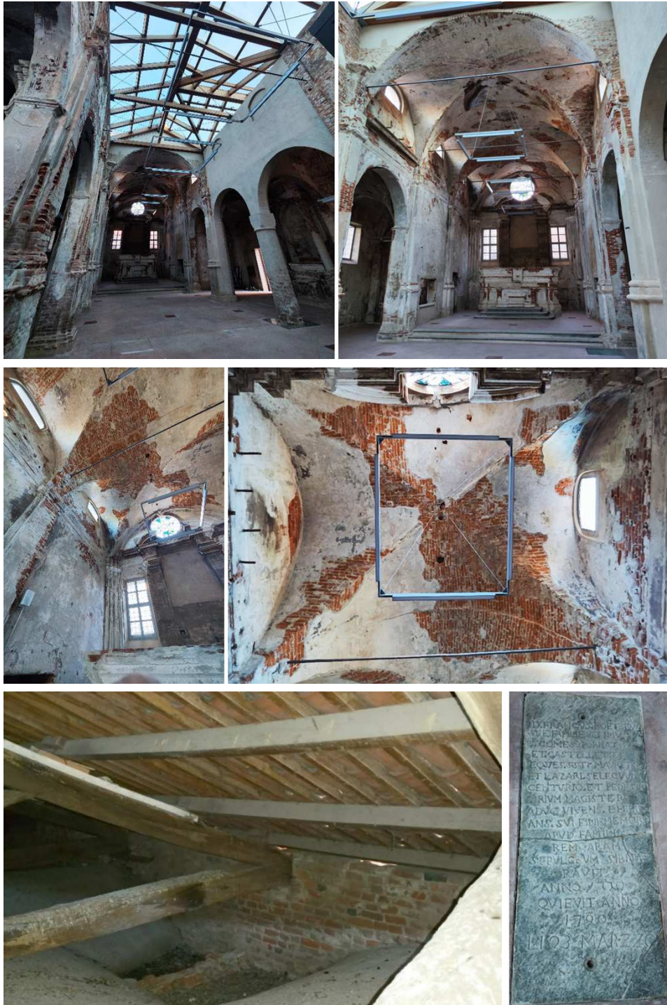
Figure 61 - Sequences of images of the central nave of the church showing the texture of the cross-vault and a view from the extrados.
