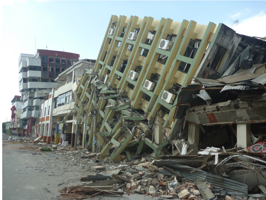
Fig. 2.1 Buildings destroyed by a 7.8 magnitude earthquake on April 16, 2016 in Ecuador. (Source: J. Lance (European Union/ECHO) [CC BY-NC-ND 2.0 ( http://creativecommons.org/licenses/by-nc-nd/2.0/ )], via Flickr; http://www.flickr.com/photos/eu_echo/26571713861 )
