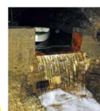
Spillway for underground collector flow rate monitoring
