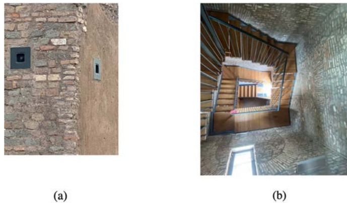
Figure 2: (a) The steel frame, (b) the spiral staircase.
