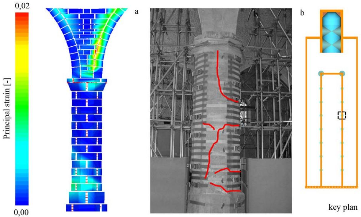
Figure 11: Comparison between the analysis results (a) and actual distribution of cracks observed after the 2009 L'Aquila earthquake (b) in one of the nave's columns.
