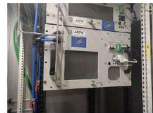
Figure 2 Installed electrolyser at ZEM module
