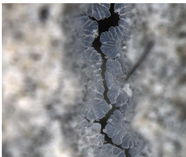
Fig. 9. Optical micrographs of a detail of a repaired zone.
