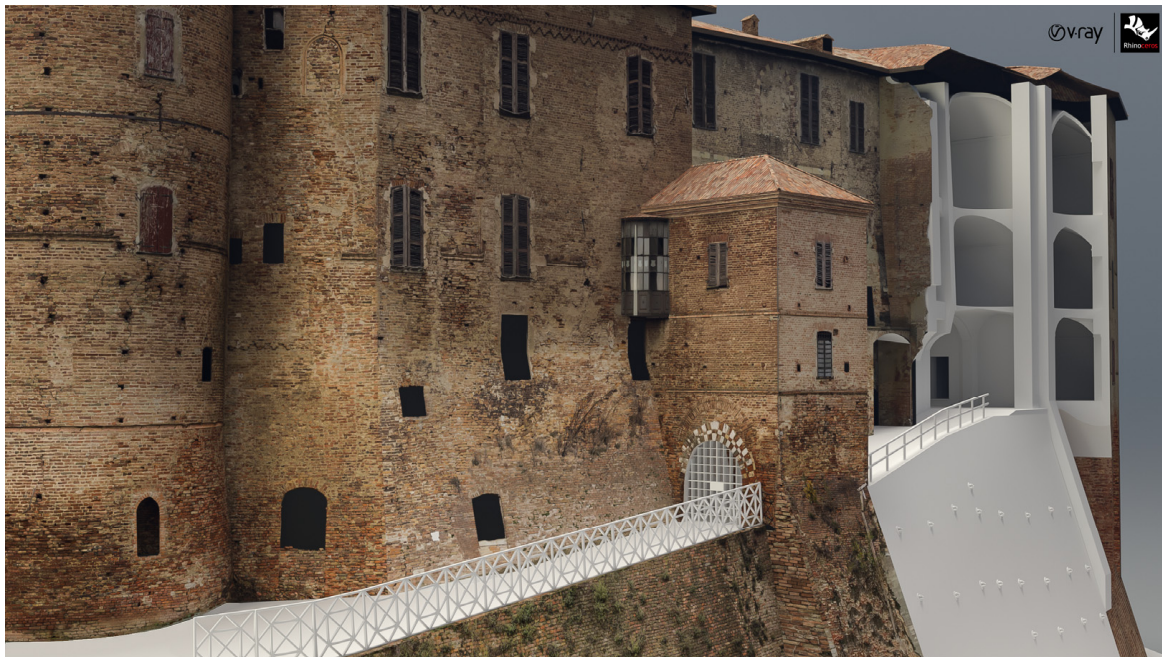
Figure 22. Textures and orthophotos mapped on the NURBS model of the castle related to the actual situation: the collapsed area on the south side.
