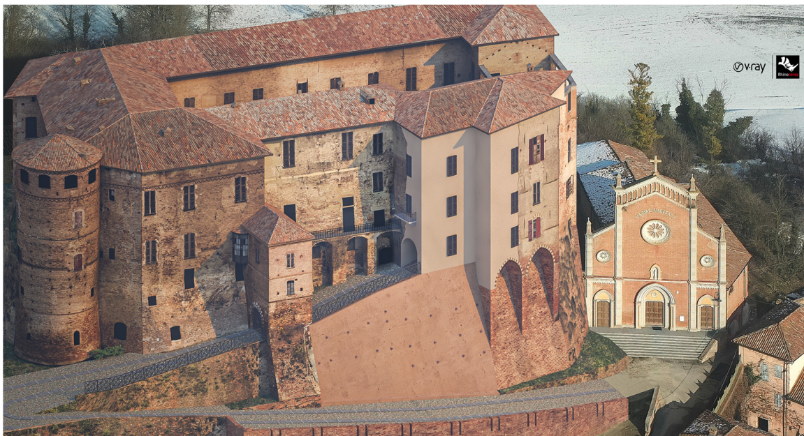
Figure 27. The 3D-rendered model proposed for reconstructing the collapsed area: modelled with Rhinoceros and V-Ray. Isometric view of the south front of the castle.
