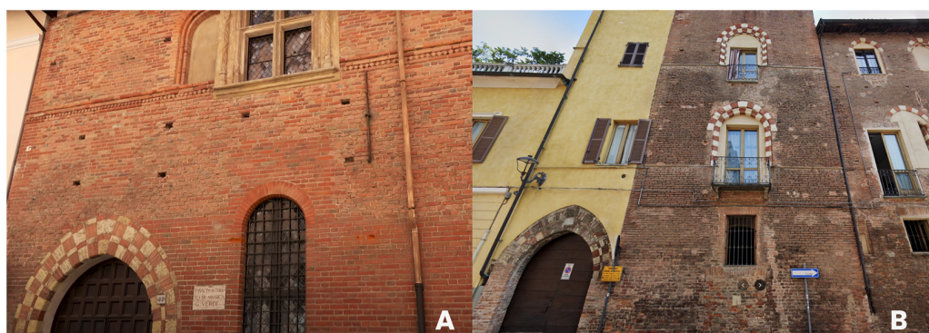
Figure 16. Comparisons on bichrome pointed arches related to doors and windows (ogival): (A) Verasis-Asinari Palace; (B) Roero Monteu Tower. From Google Street View.
