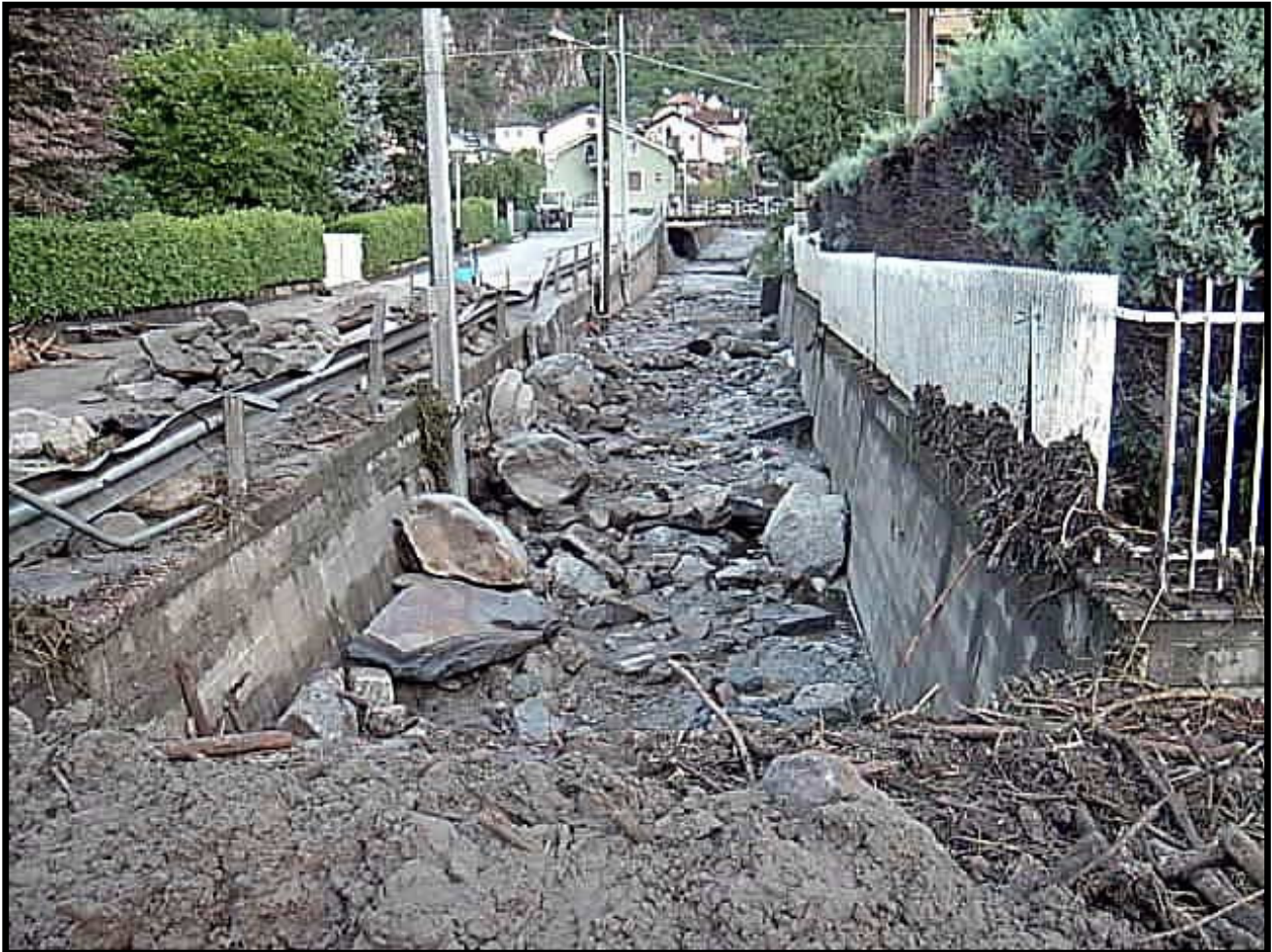
Figure 2. Debris flow deposit in channel bed.
