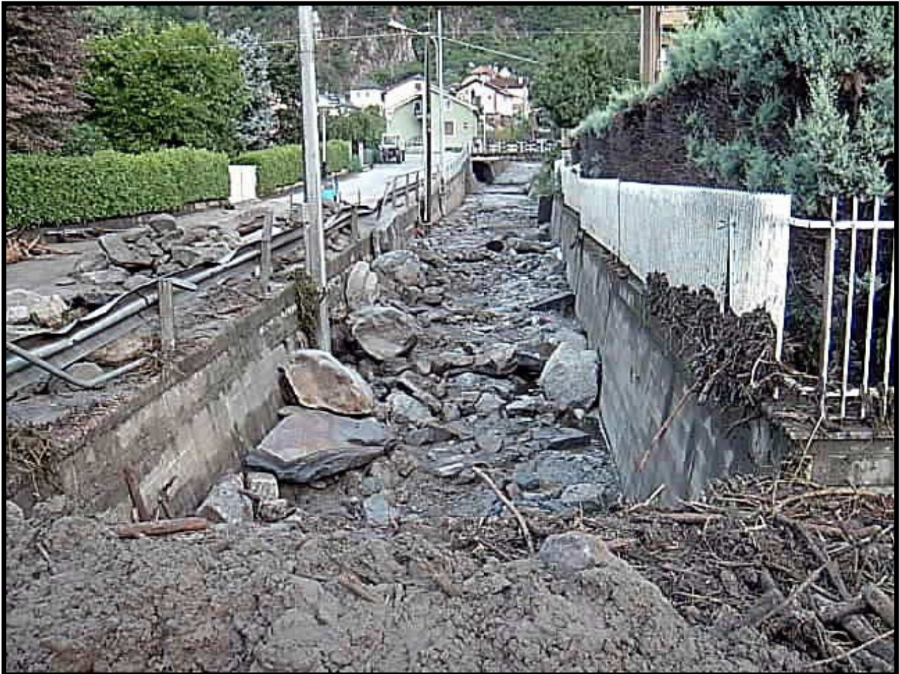
Figure 2. Debris flow deposit in channel bed.
