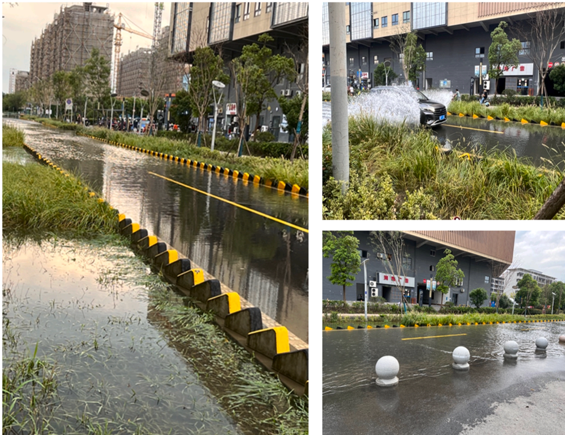
Fig. 3. Flood occurrence after typhoon Muifa on 13 September and inundation of the swale. Photo source: Lingwen Lu (approved to use the photos). (For interpretation of the references to color in this figure legend, the reader is referred to the web version of this article.)
