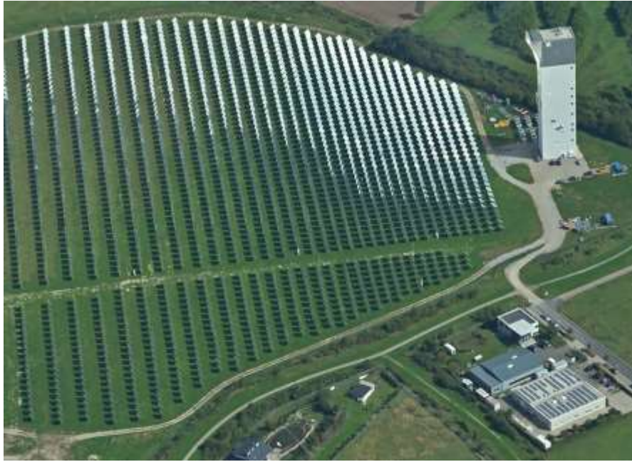
Figure 8-3: Example of a CSP plant based on solar tower concept [185]
