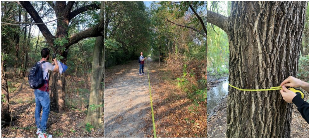
Figure 3.11: Some photos from the site inspection (September 2021).
