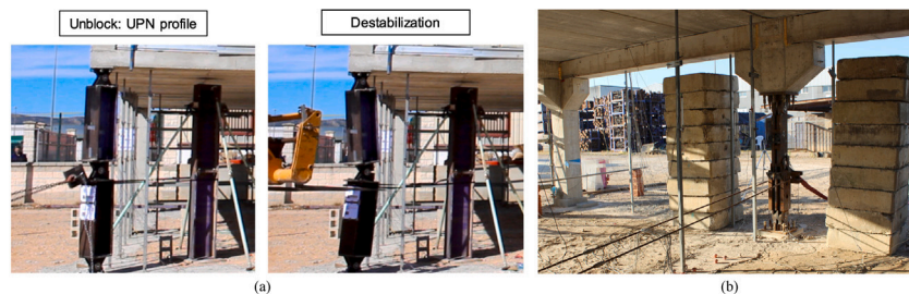
Fig. 13. Dynamic column removal in dummy column assemblies (a) pushing by slight destabilization of the column using a forklift, as reported in [30] and (b) pulling, the cables were connected to a hydraulic jack (test performed at Universitat Politècnica de València [57]).
