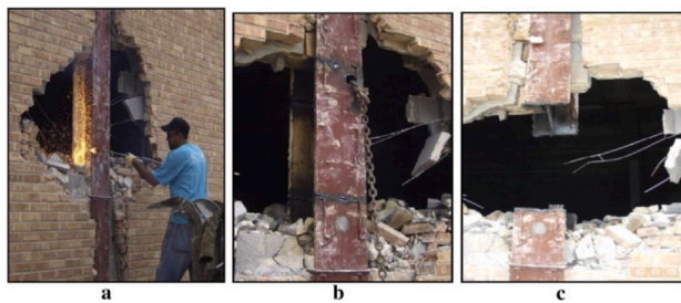
Fig. 10. Dynamic column removal in existing steel frame building; (a) torching of the removed column, (b) column ready to be pulled out, and (c) removal of the column, as reported in [56].
