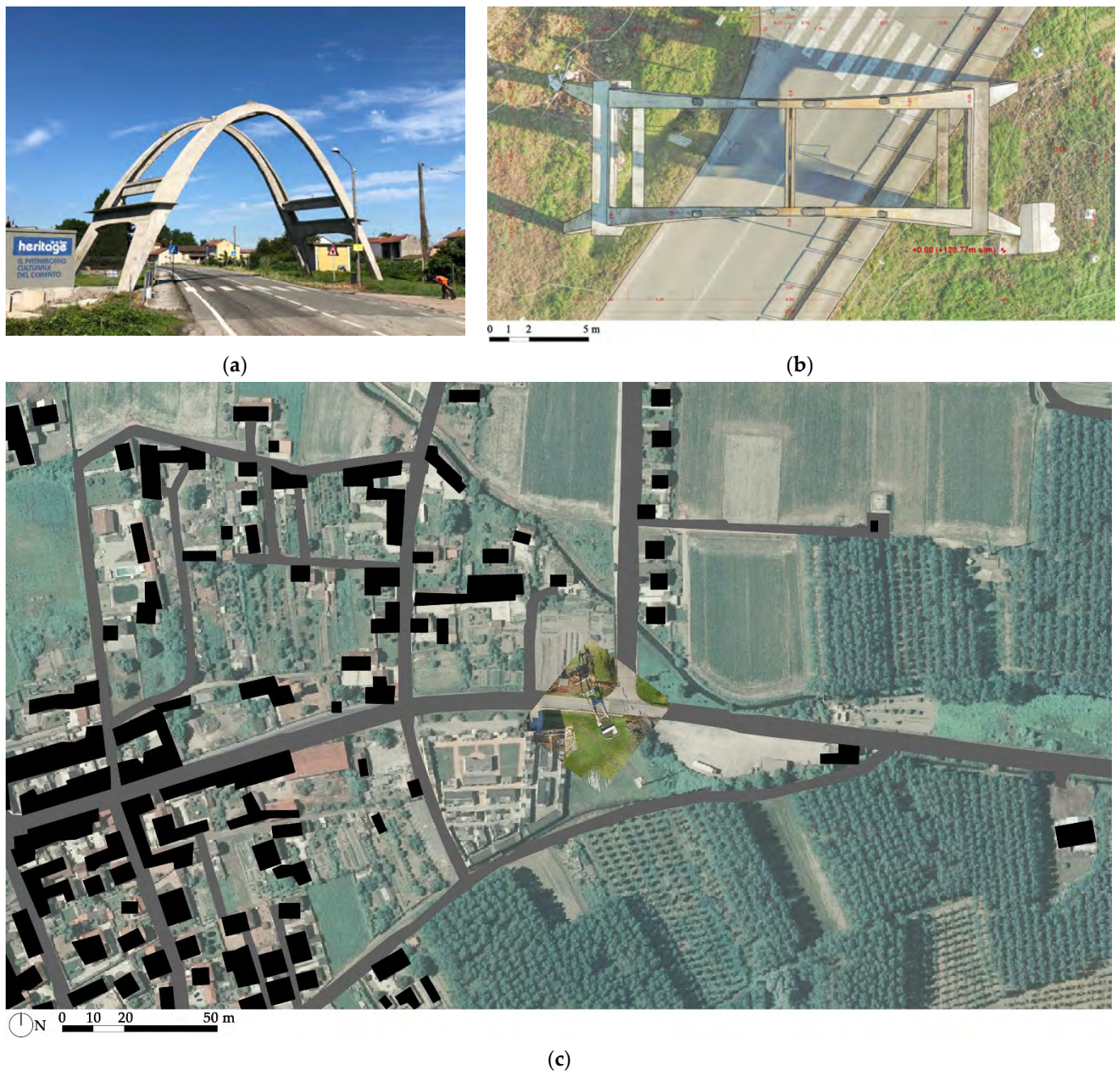
Figure 1. (a) Current view of Morano's Arch; (b) plan view from a UAV-photogrammetry-based orthophoto; (c) UAV orthophoto (0.005 m) overlaid on a regional orthophoto (GSD: 0.5 m), with buildings (black) and roads (grey) from a regional CTRN.
