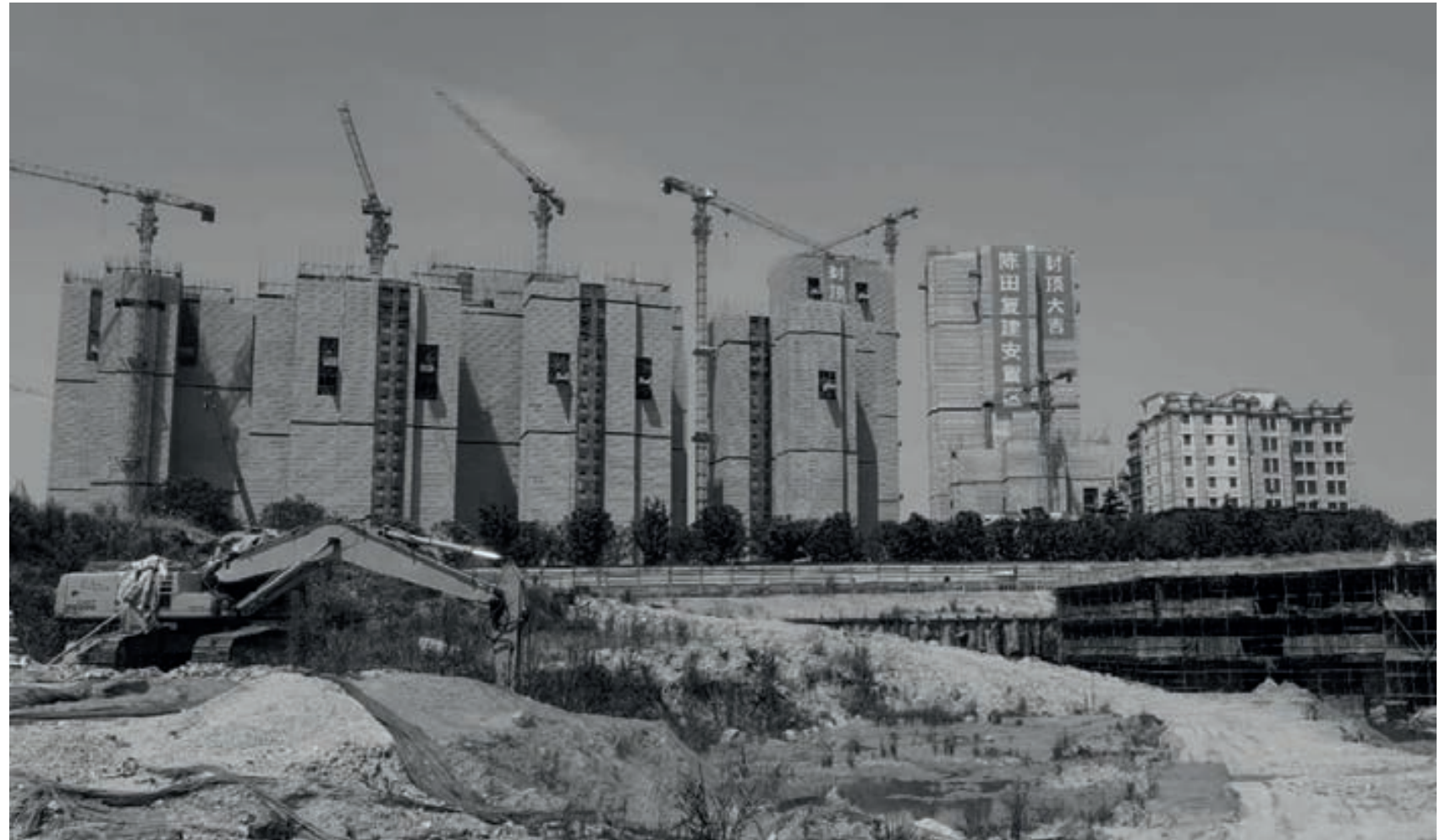
Renovated houses for urban villagers © Shan Jia
