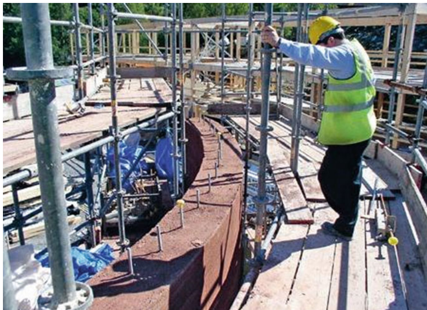
Fig. 33.7 Construction of the lecture theatre of the WISE at the Centre for Alternative Technology. The attractive load-bearing rammed-earth walls, 500 mm thick, are pneumatically tamped and left unfinished on both faces. Photo Pat Borer
