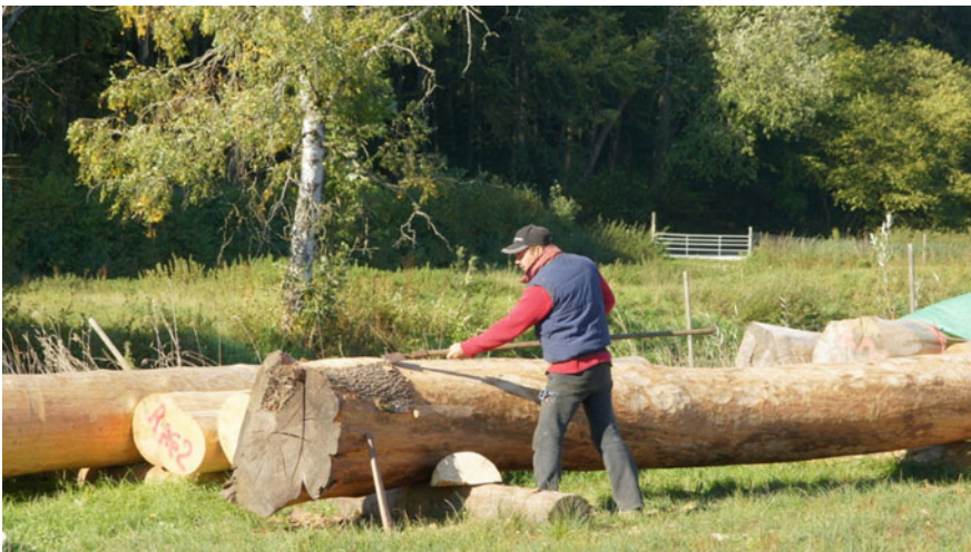
Fig. 33.3 Manual debarking of trees at Biotal site. Untreated logs are used as structural columns in the building. Photo Christoph Bosch
