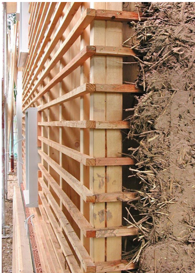
Fig. 33.6 Light-earth external skin applied onto battens in a new house in Darmstadt. Photo Franz Volhard
