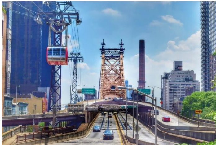
Figure 39-Picture of the aerial to-and-fro ropeway “Roosevelt Island” in New York City- NY
