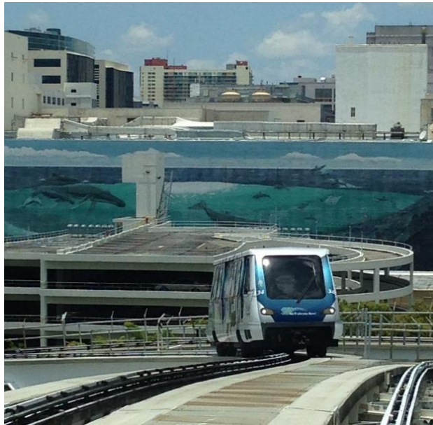
Figure 36-Picture of the Metro Mover installation in Miami-Florida
