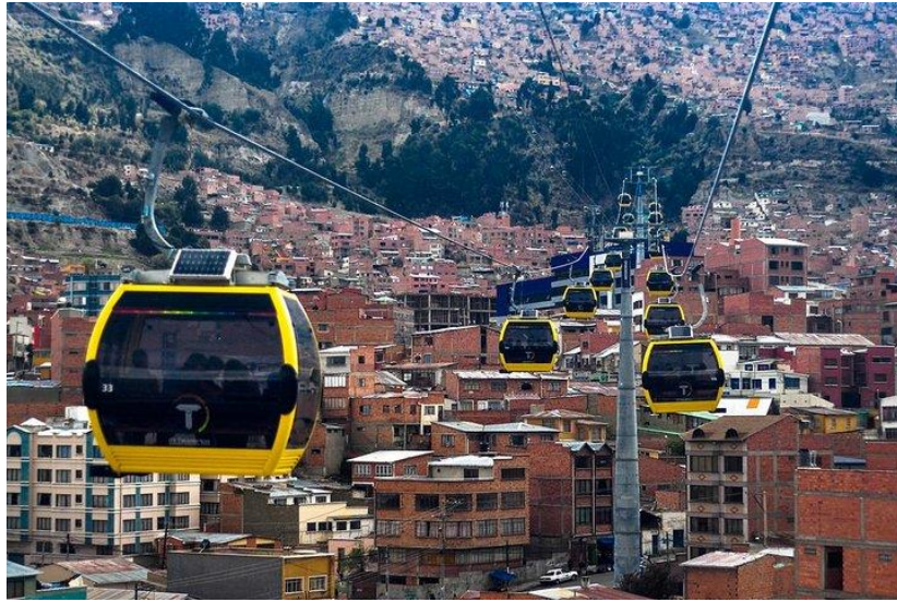
Figure 18-Picture of a line of “Teleferico” installation in La Paz- Bolivia
