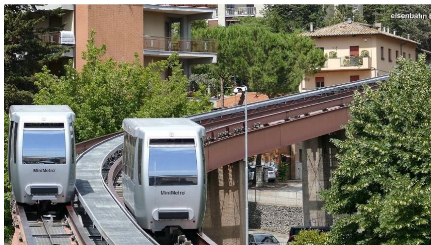
Figure 37-Picture of the Mini Metro installation in Perugia (Italy)
