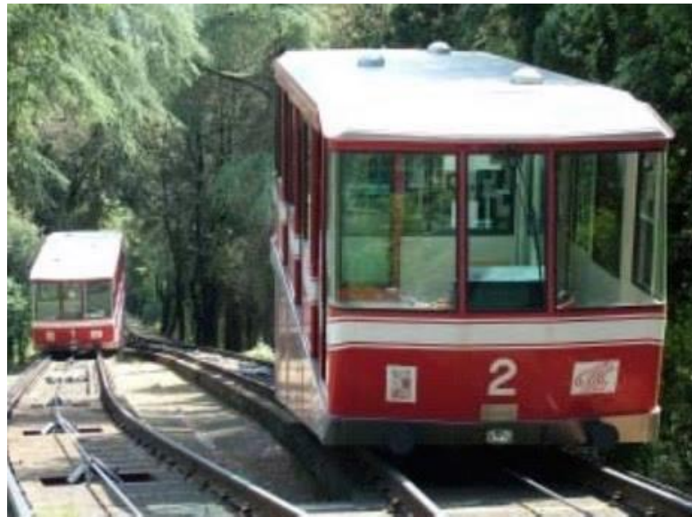
Figure 32-Picture of a funicular ropeway, in the switch area
