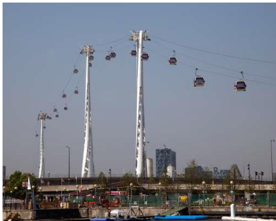
Figure 113-Picture of the towers of the traditional monocable gondola “Emirates airline” in London- UK
