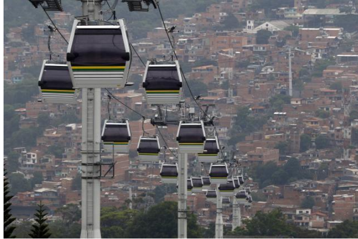
Figure 17-Picture of a line of “Metrocable” installation in Medellín- Colombia
