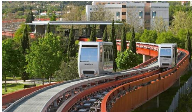
Figure 22-Picture of the line of Minimetro mobility system in Perugia
