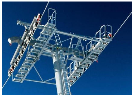
Figure 46-Picture of a compression tower
