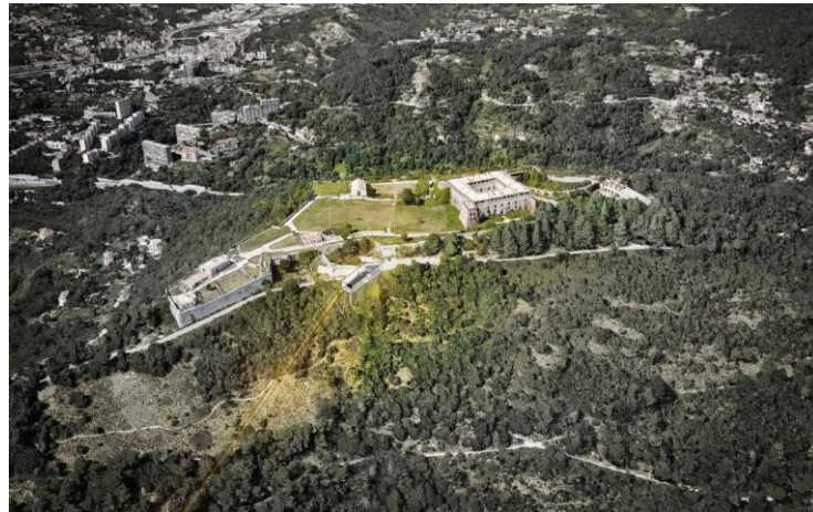
Figure 116-Area of installation of the upstream station in Forte Begato
