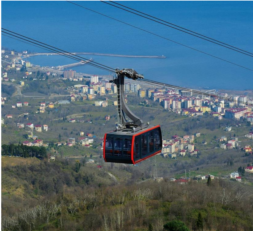
Figure 38-Picture of an aerial to-and-fro ropeway
