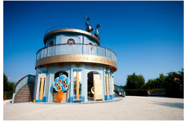
Figure 3. The Fantacasio building in Venaria Reale (Torino, Italy). Source: https://lavenaria.it/en/activities/fantacasio
