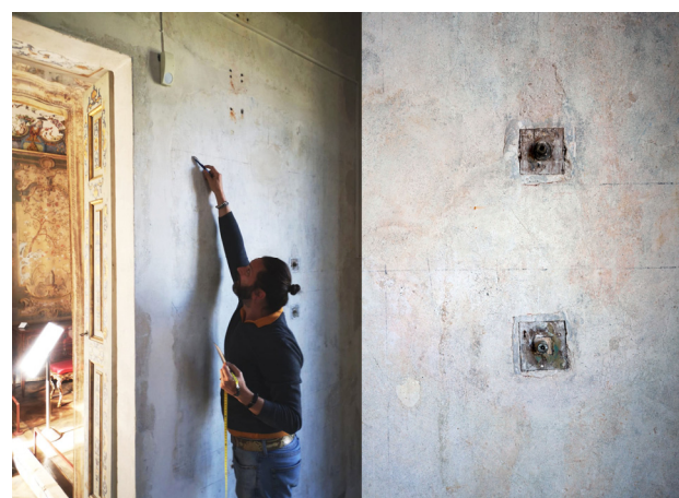
Figure 9. Identification of the geometric pattern for assembling the furniture and iron clasps in the cabinet of Villa della Regina (Photo: E. Pupi).
