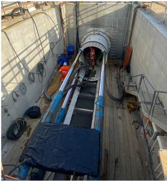
Fig. 2 The system of pushing the elements of the reinforced concrete pipeline through hydraulic jacks that contrast on the side walls of the thrust shaft
