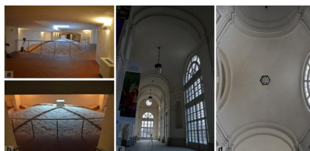
Figure 2. a-b) Vault extrados; c) ground floor space; d) vault intrados.
