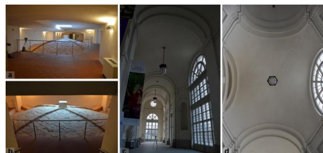
Figure 2. a-b) Vault extrados; c) ground floor space; d) vault intrados.
