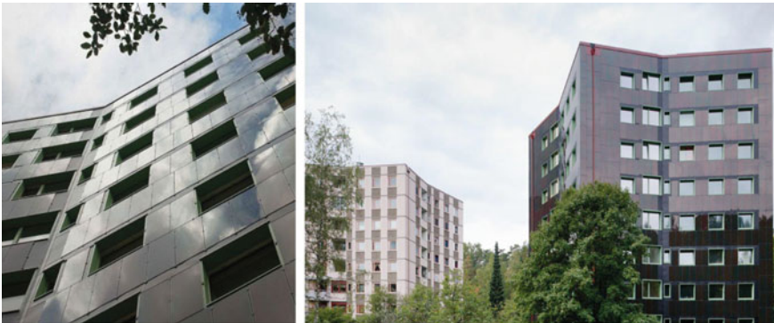
Fig. 29.13 Renovation of Stacken apartment building
