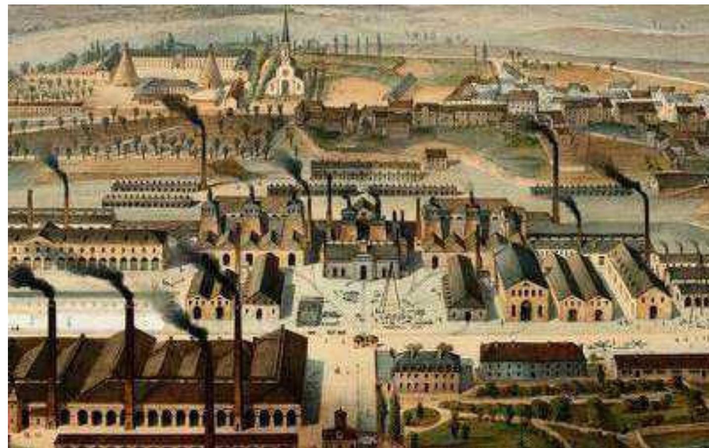
Fig.2. Le Creusot, as one of complexes that applied the new disciplinary guidelines.
