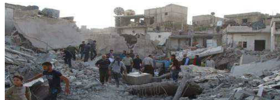
Fig.8. Destroyed concrete buildings in Aleppo, Syria (Aljazeera, 2016).
