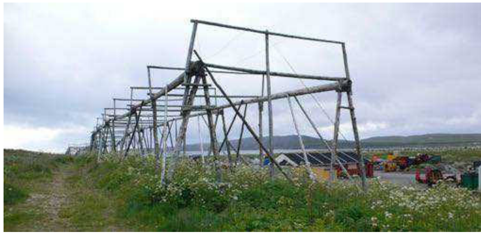
Fig.5. Vardø's structure for drying fish. Photograph: Susana Ventura, 2014.
