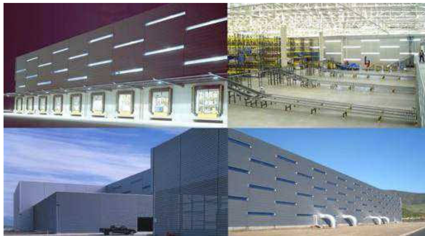
Fig.7. Distribution Center FASA / GH+A | Guillermo Hevia. Source: G. Hevia.
