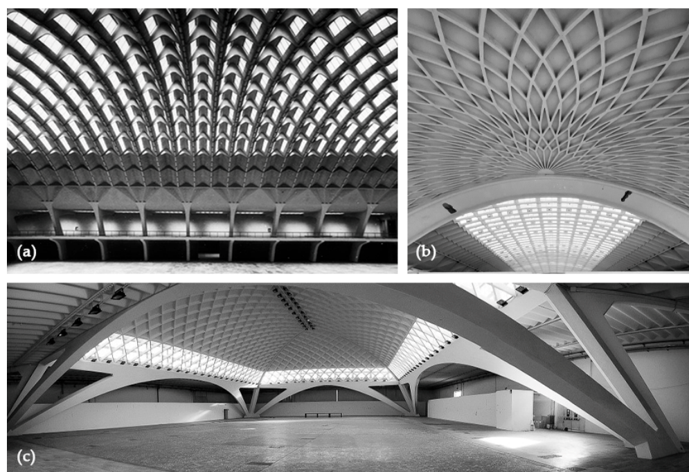
Figure 1. The wide and impressive reinforced concrete vaulted structures of the Nervi’s halls (photos from the archive of the conservation plan—Politecnico di Torino): (a) the wide undulated vault form pavillon B; (b) the semi-dome ribbed vault of the exedra, pavillon B; (c) the inclined arches from C pavillon.
