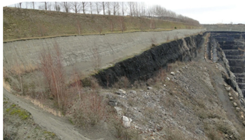
Figure 4. Layers of grey silty sand forming the overburden at a large open pit quarry for limestone; a layer of dark limestone is visible in between the burden and rock benches (credits C. Oggeri).
