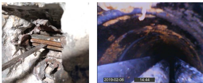
Fig. 20. Visual inspection of post-tensioning tendons in a rib (left), and endoscopy inspection inside a duct of the rib (right) (MASTRLAB 2019).
