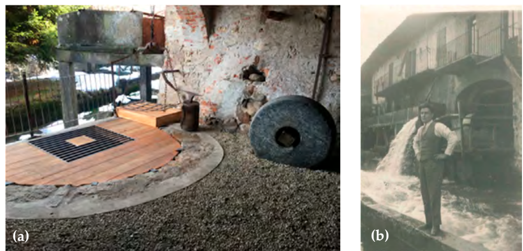
Figure 10. The hemp roller mill; (a) The position of the old vertical axis water wheel; (b) the hemp roller mill photo from the 1930s on the right, under the arch.
