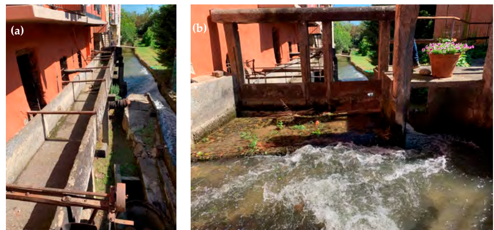
Figure 15. (a) The flume; (b) the water wheel flume gate (left) and the hydraulic trompe flume gate (center).
