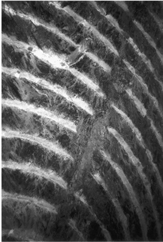
Figure 2.66 Grooves left on the tunnel face by disc cutters.
