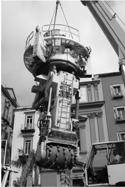
Figure 2.136 Detail of the boring unit.
