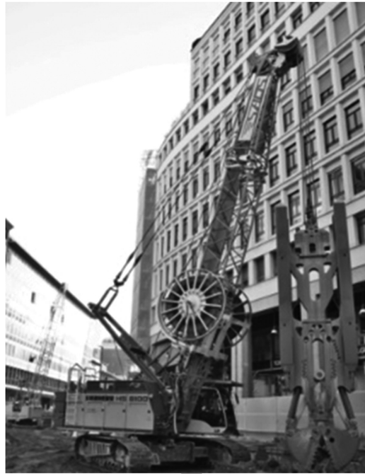
Figure 2.143 Picture of LWN HSG 5–18 working in the Milan metro.
