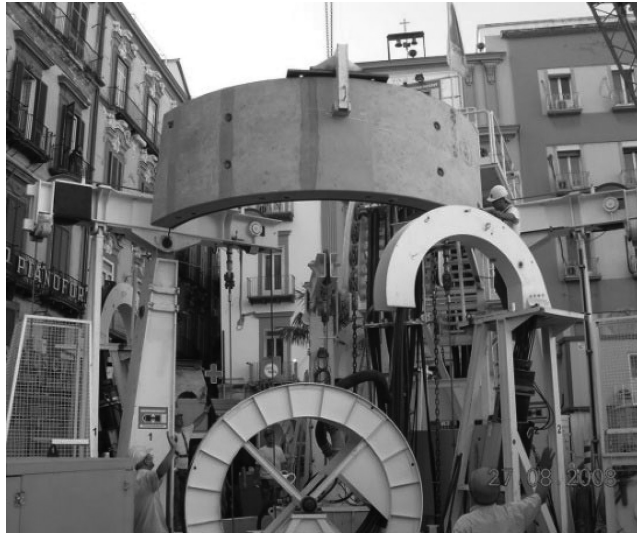
Figure 2.137 Installation of the lining segments at the top of the shaft.
