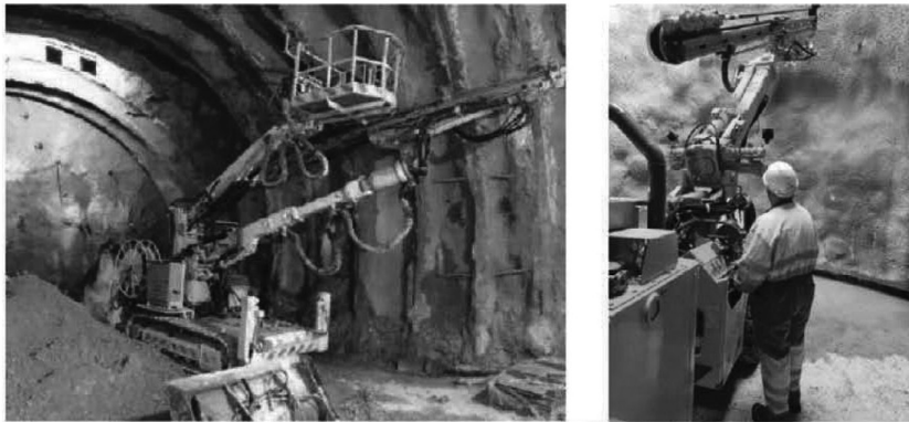
Figure 2.11 Example of customised jumbos for special applications: ground reinforcement and bolting, in Grand Paris tunnels. (Courtesy of Robodrill.)
