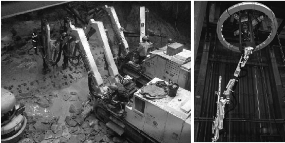
Figure 2.128 Example of shaft drilling jumbos. (Courtesy of Robodrill.)
