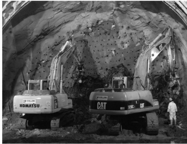
Figure 2.21 Example of a drill and split tunnel face with two machines work in parallel.
