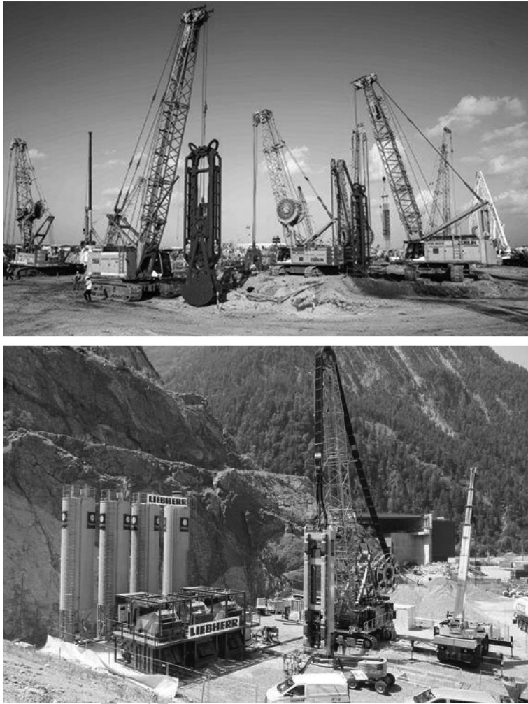
Figure 2.140 Grab excavation in port said and trench cutter in a mountains side.
