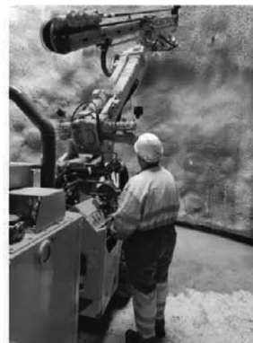
Figure 2.11 Example of customised jumbos for special applications: ground reinforcement and bolting, in Grand Paris tunnels. (Courtesy of Robodrill.)
