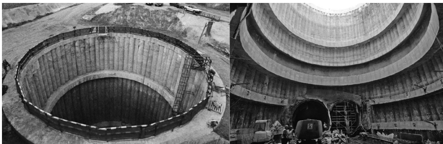
Figure 2.156 Secant piles shaft (a) and mixed secant and tangential piles shaft (b).
