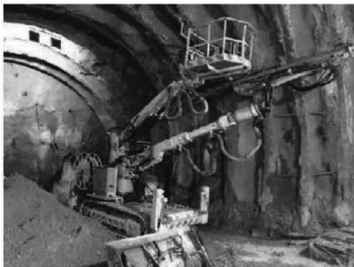
Figure 2.11 Example of customised jumbos for special applications: ground reinforcement and bolting, in Grand Paris tunnels. (Courtesy of Robodrill.)
