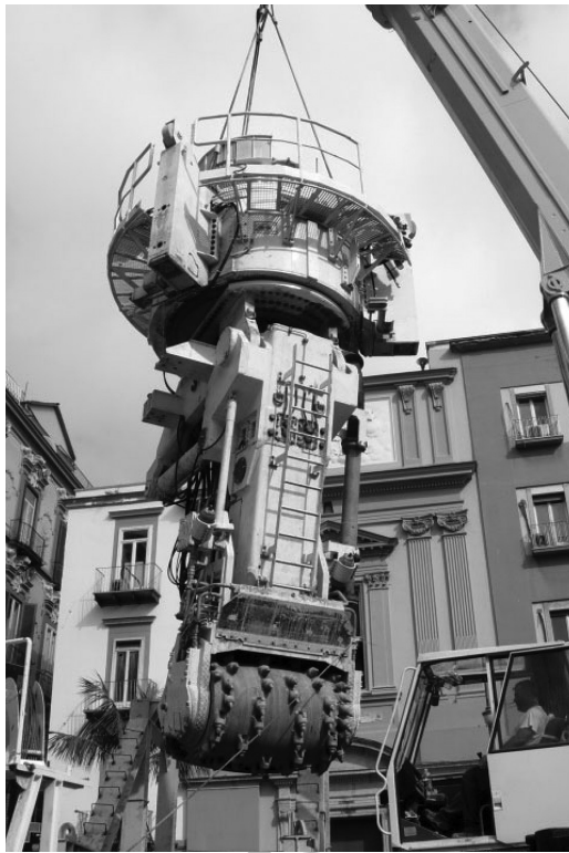
Figure 2.136 Detail of the boring unit.
