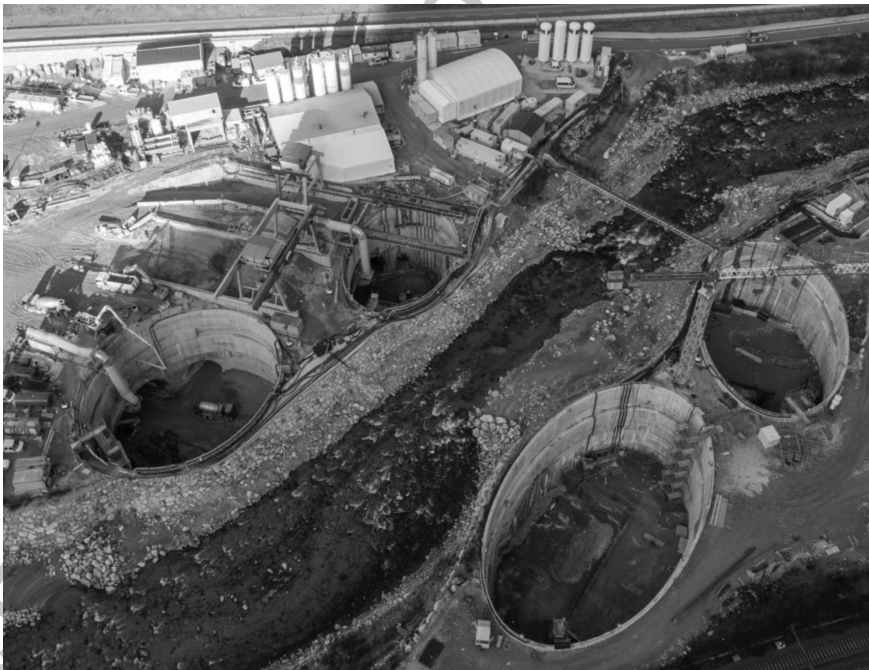
Figure 2.125 Picture of the construction phase of the four shafts near the Isarco River. (Courtesy of BBT SE.)
