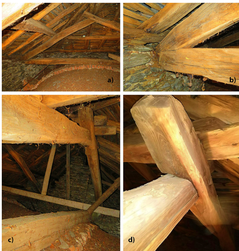
Fig. 5. (a) North truss; (b) detail of the tie beam-rafters connection, in evident degradation inside the masonry support; (c) tie beam rests on the extrados of the vaults; (d) detail of a half-lap coupling connection.
