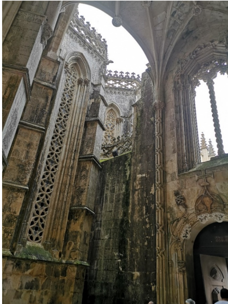
Figure 4.1. Bio-degradation on the inner wall of the “imperfect chapels” of the Batalha Monastery.
