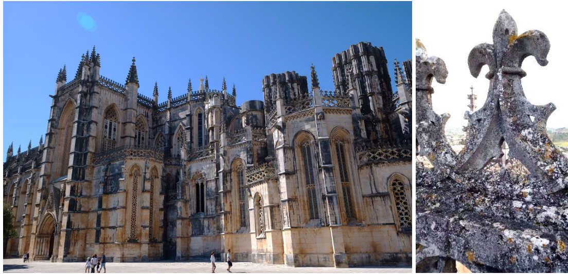
Figure 3.1. (left) The external wall of Batalha Monastery, covered by dark brown/gray biofilms and crusts; (right) Balustrade on the roof of the monastery showing thick biofilms and lichenous crusts.
