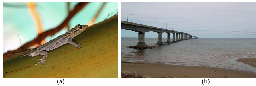
Figure 2. Compartmentalization concept; (a) nature: a survived white-headed dwarf gecko with tail lost due to autotomy [33] (taken by Muhammad Mahdi Karim, with no modification under GNU Free Documentation License, Version 1.2) and (b) engineering: Confederation Bridge in which a limited collapse is accepted to ensure the structural robustness [34] (with no modification under Creative Commons Attribution 2.0 Generic license ( https://creativecommons.org/licenses/by/2.0/ , accessed on 2 February 2023)).
