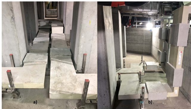
FIGURE 23. Sections of the closure of loops A and C: a) path under the furnace; b) ascent towards the busbar ducts.
