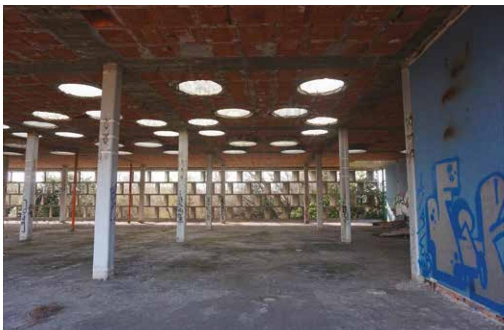
the buildings are significantly resilient thanks to their concrete structures and façades, but the reuse thereof would require analogic reconstruction of the glass casing, partitions and technological systems performance for thermal and acoustic comfort, consolidation and surface restoration works of concrete, while checking also for static safety.
