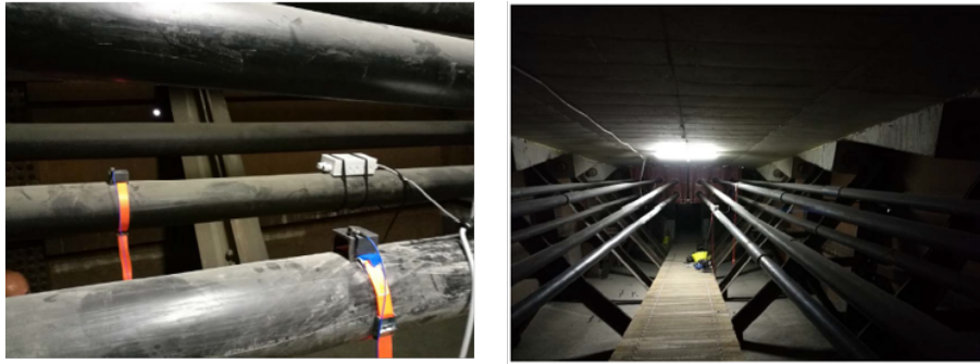
Figure 3: Internal installation of the sensors on the prestressed tendons.
