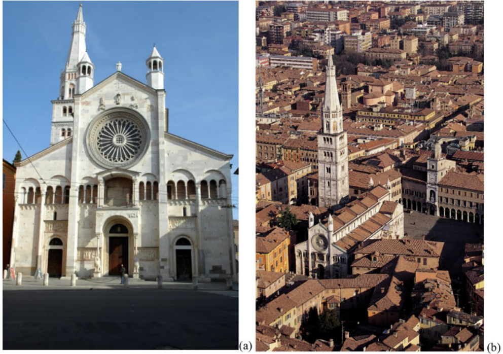
Figure 1. (a) The façade of the Cathedral; (b) Aerial view of the Cathedral and the Ghirlandina Tower.
