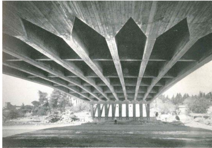
Figure 34: Via Olimpica overpass, Rome, 1958-1959: bottom view (Boaga, 1984)
