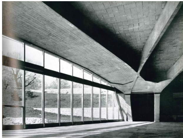
Figure 52: View of the closed stiffening box system between for the external pair of ribs (Boaga, 1984)
