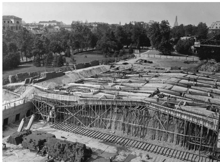
Figure 59: View of the construction site of Pavilion V of Turin Exhibition Center, 1959
