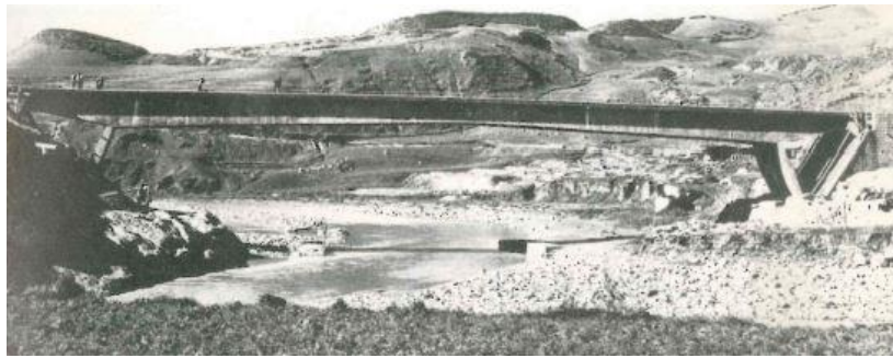
Figure 32: Bridge over the Cerami, Enna, 1953-1954: general view (Boaga, 1984)
