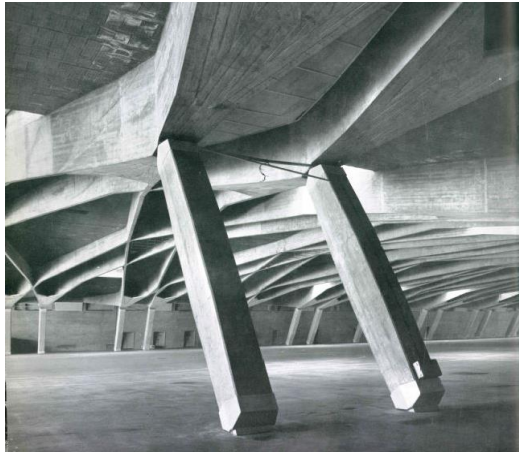
Figure 12: Underground exhibition hall in Turin, Italy
