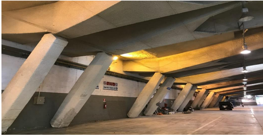
Figure 58: Internal view of the pavilion after the insertion of the fire walls
