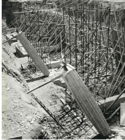
Figure 61: Photography of Pavilion V construction site: longer strut beams
