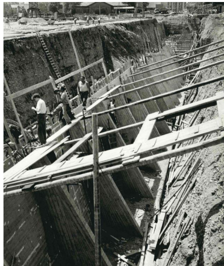
Figure 62: Photography of Pavilion V construction site: retaining walls
