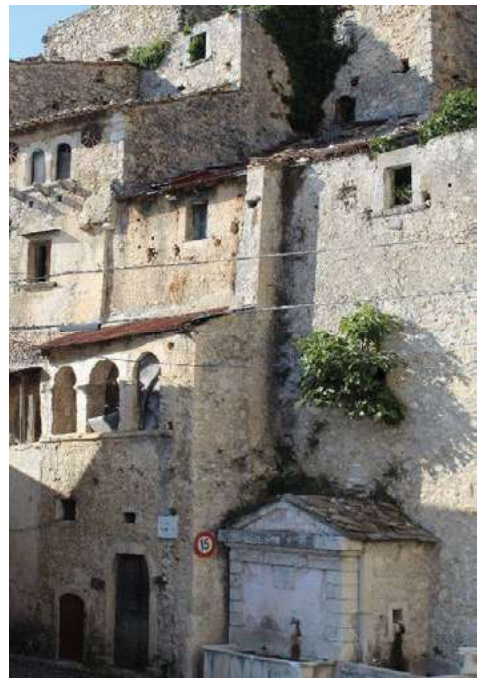
Fig. 4. Buildings of Pesche's historic centre (2021).
