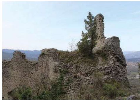
Fig. 7. External view of the keep (2021).
