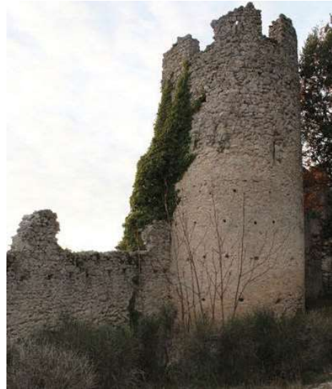
Fig. 13. Central tower with circular holes (2021).
