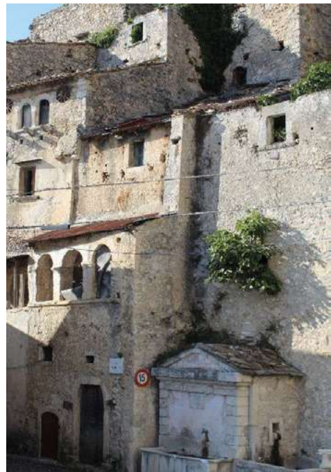
Fig. 4. Buildings of Pesche's historic centre (2021).
