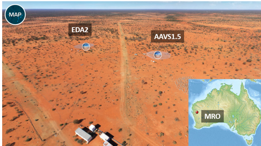
Fig. 3.1 Aerial view of the AAVS1.5 and EDA2 stations at the MRO site. Picture from https://virtualtours-external.csiro.au/MRO/ .
