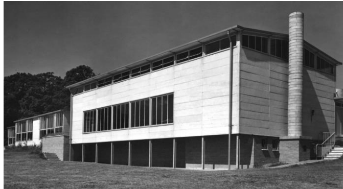
Fig. 5: Essendon Primary School, Hertfordshire: an early example of prefabrication in school buildings, made of light steel-framed system [13]
