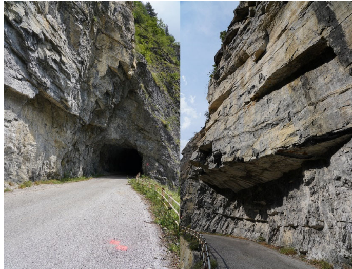
Figure 1. Photographs of the rock walls under study.
