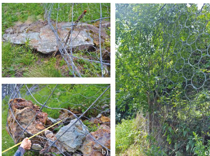
Fig. 4 – Frequent observed damages: voids at the foot of the barrier (a), debris/blocks/notches in the net (b), and elements limiting the deformation capacity of the barrier (c).
