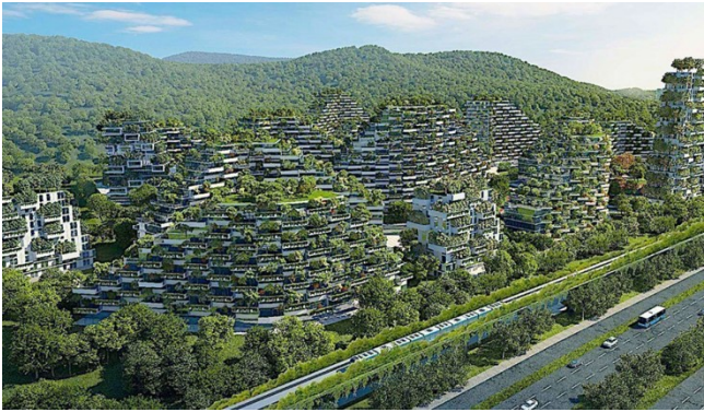
Fig. 1. The Forest City in the Chinese city of Liuzhou, designed by Stefano Boeri architecture studio.
