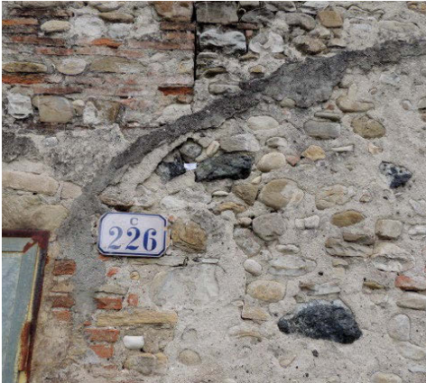
Fig. 8. Particular of masonry made of river pebbles and bricks laid with abundant mortar (Source: Fratini).
