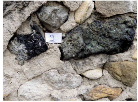
Fig. 10. Analysed bedding mortar (Source: Fratini).
