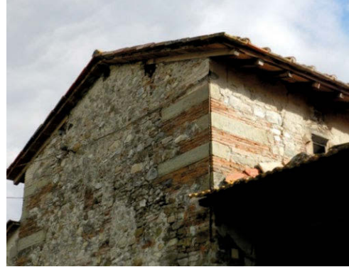
Fig. 5. Detail of the masonry at the corner of a drying room (Source: Mattone).
