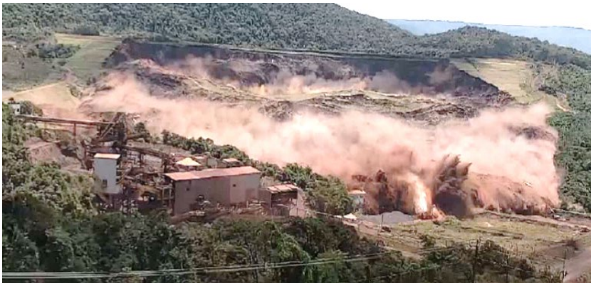
Fig. 1: The collapse of Feijão tailing dam - Brazil – 2019 ([8]).
