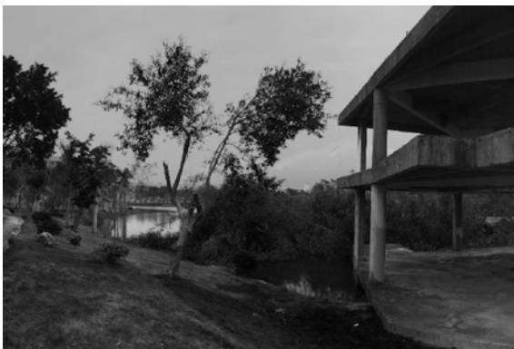
Figure 3.35 Difference of ground level in School of Future Design of BNU ©THAD
