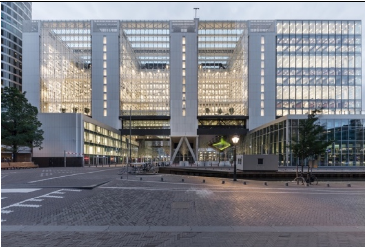
Figure 2.1 Renovation of Rijnstraat 8 (photo by Delfino Sisto Legnani and Marco Cappelletti)
