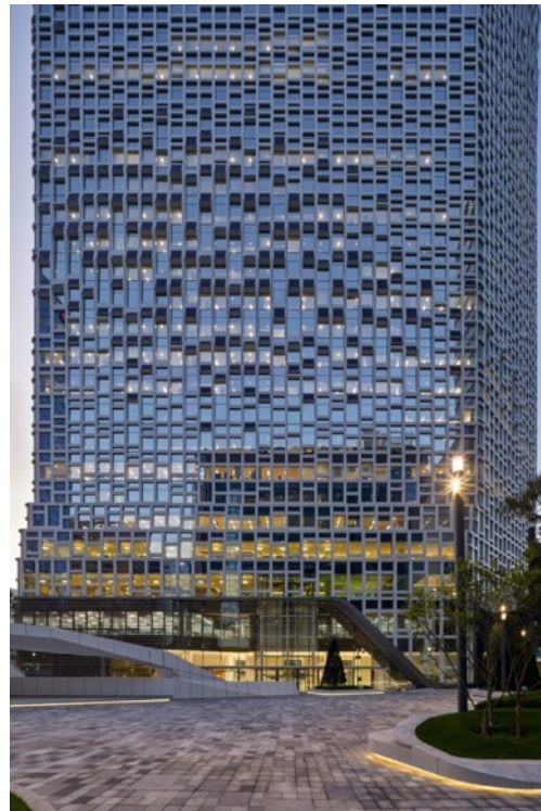
Figure 2.16 Hanhua Headquarter after renovation ©UN studio
