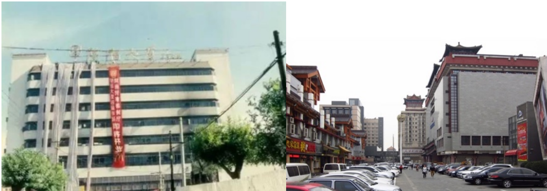
Figure 1.3 Longfu Building renovated for many times. Left: Longfu Building in 1990s ( https://www.sohu.com/a/79587887_407820 ); Right: Longfu Building in 2012 (photo by Zhou Kai)
