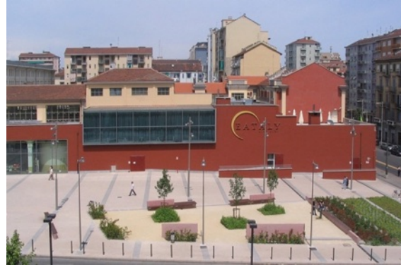
Figure 3.34 Paving of plaza outside Eataly © Negozio Blu Architetti
