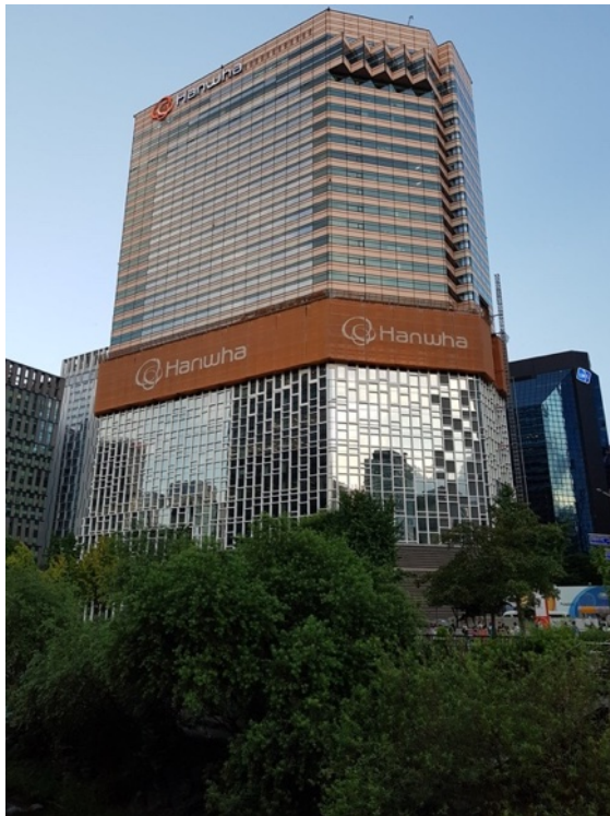
Figure 2.15 Hanhua Headquarter in renovation https://skyrisecities.com/forum
