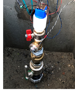
Fig. 5: Picture of the actuator mounted onto the pipe.
