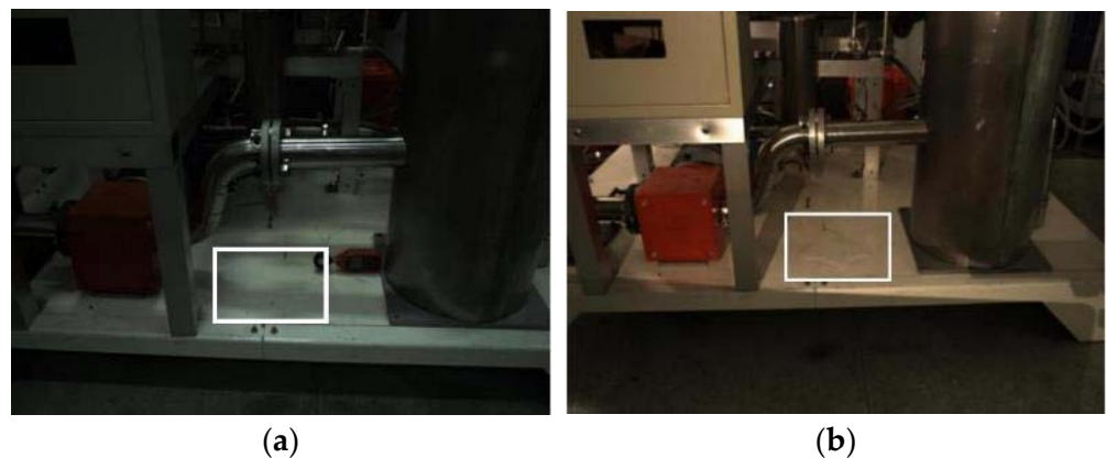
Figure 3. Difficult to detect colorless effusion (in the white box): (a) effusion feature in natural light; (b) effusion feature under LED flash light.
